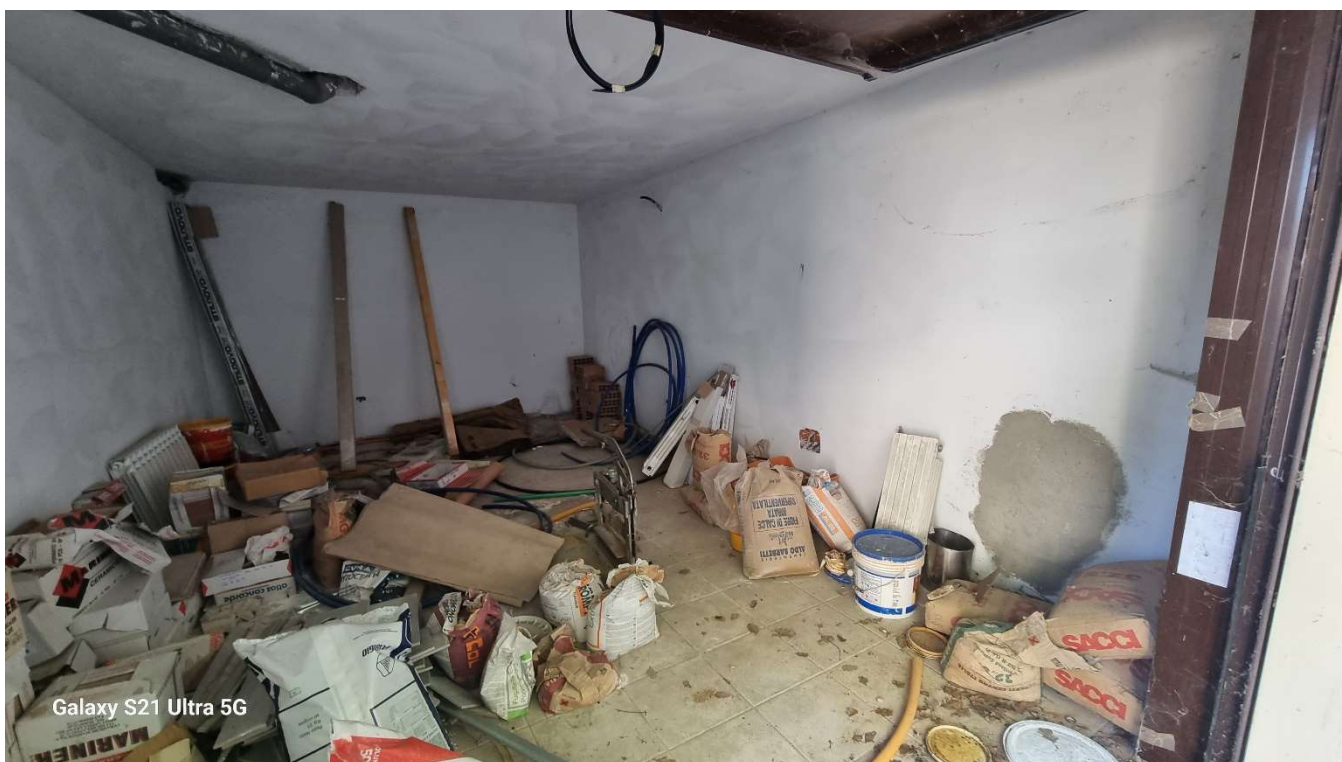
Garage – Interno locale garage
